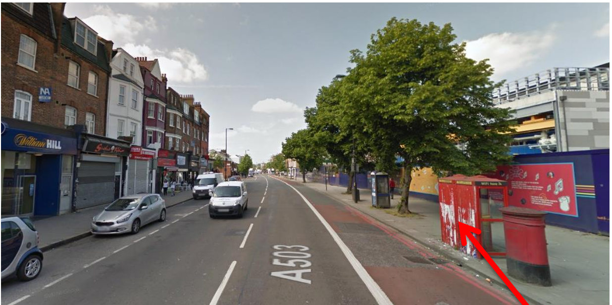
Image 2: View of the site looking west along Seven Sisters Road
